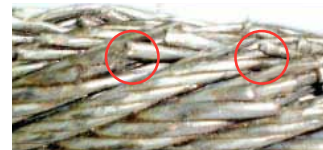
Wire Breakages at Crown
