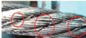
Wire Breakages at Valley
